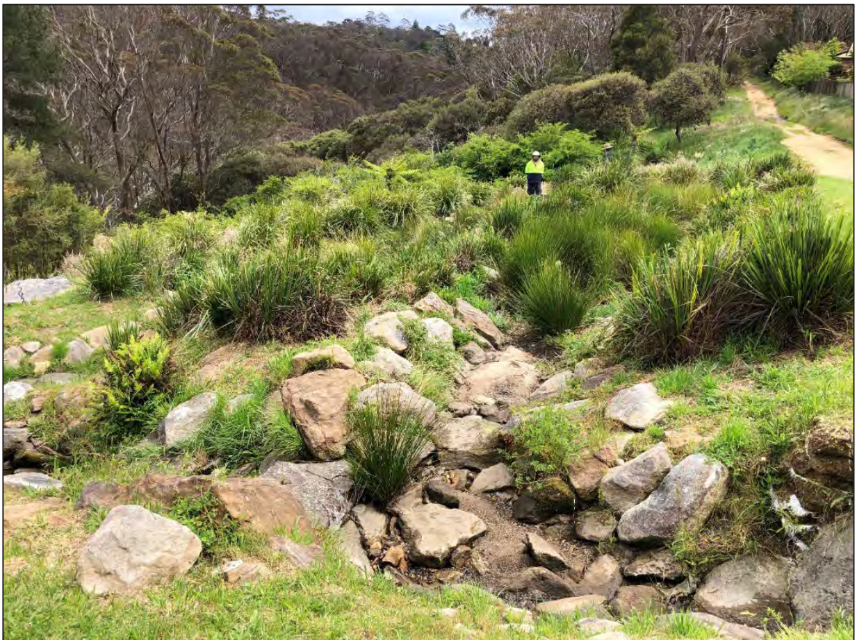
Figure 9-4: Stormwater management by Blue Mountains City Council at Leura Park
