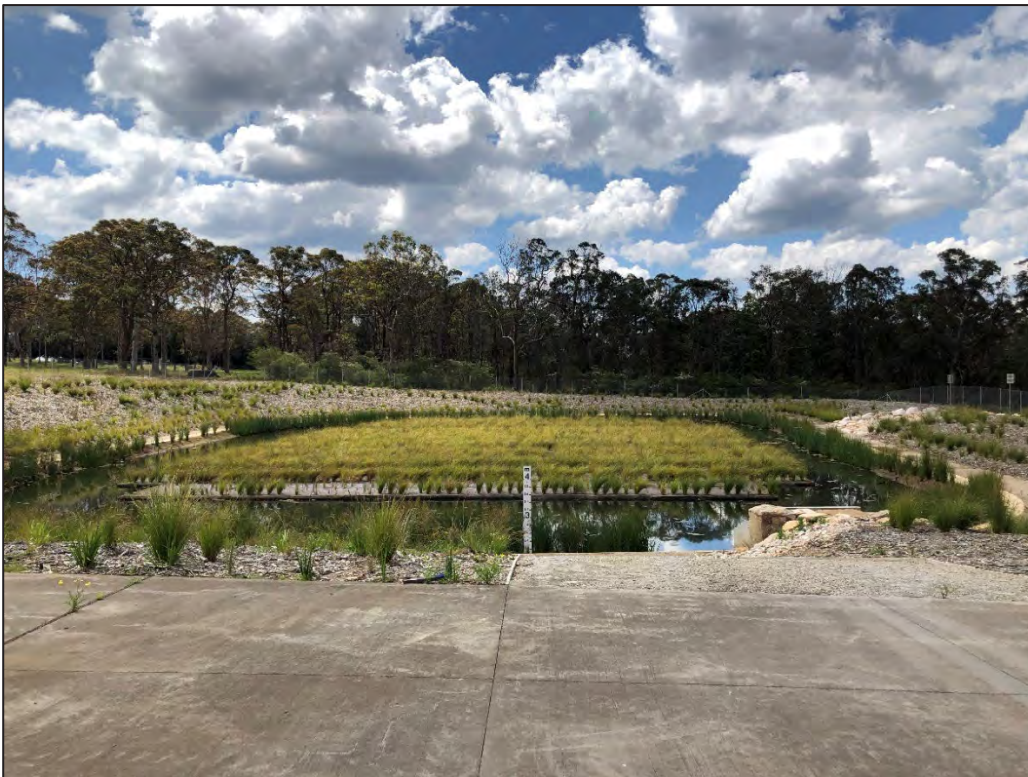
Figure 9-3: Floating wetlands installed to improve water quality at Oakdale
