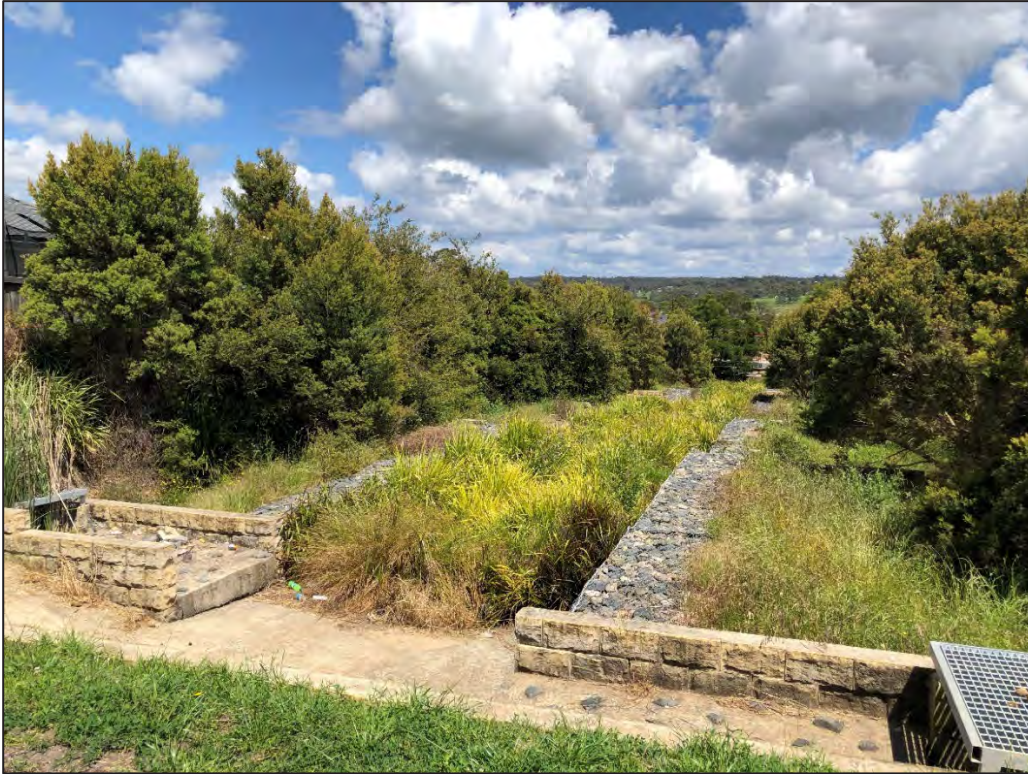
Figure 9-2: Bioretention to improve stormwater quality at The Oaks
