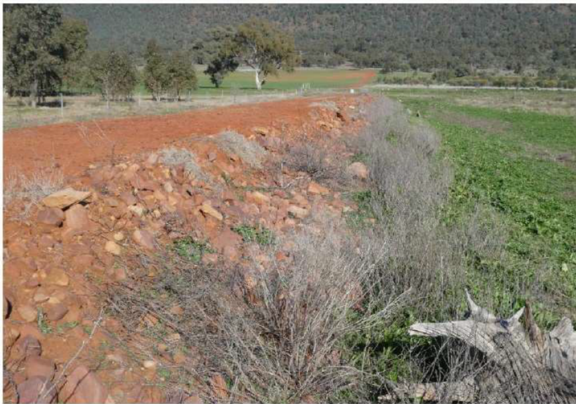
The lakeside bank of Levee L has been degraded by waves
