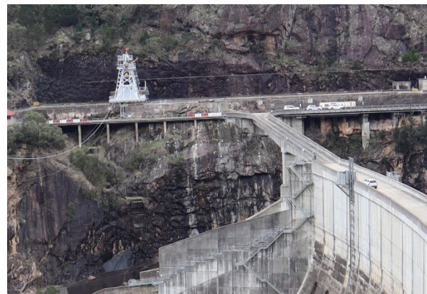
Figure 4.7 Northern head tower (viewed from southern side), with cable at left of image. (Source: WaterNSW, July 2025)
