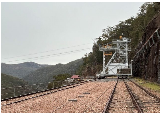
Figure 4.6 Head tower, with cable to the left. (Source: WaterNSW, July 2025)
