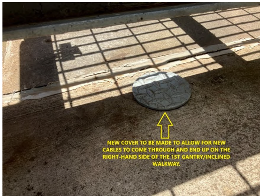
Figure 19: Cover on floor penetration from top of southern crest wall into crest chamber
