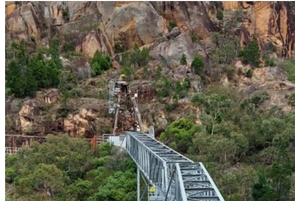
Figure 4.9 Tail tower. (Source: WaterNSW, 2023)
