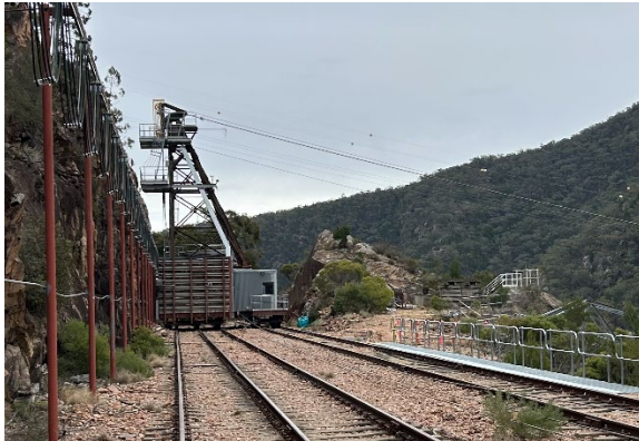
Figure 4.8 Tail tower. (Source: WaterNSW, July 2025)
