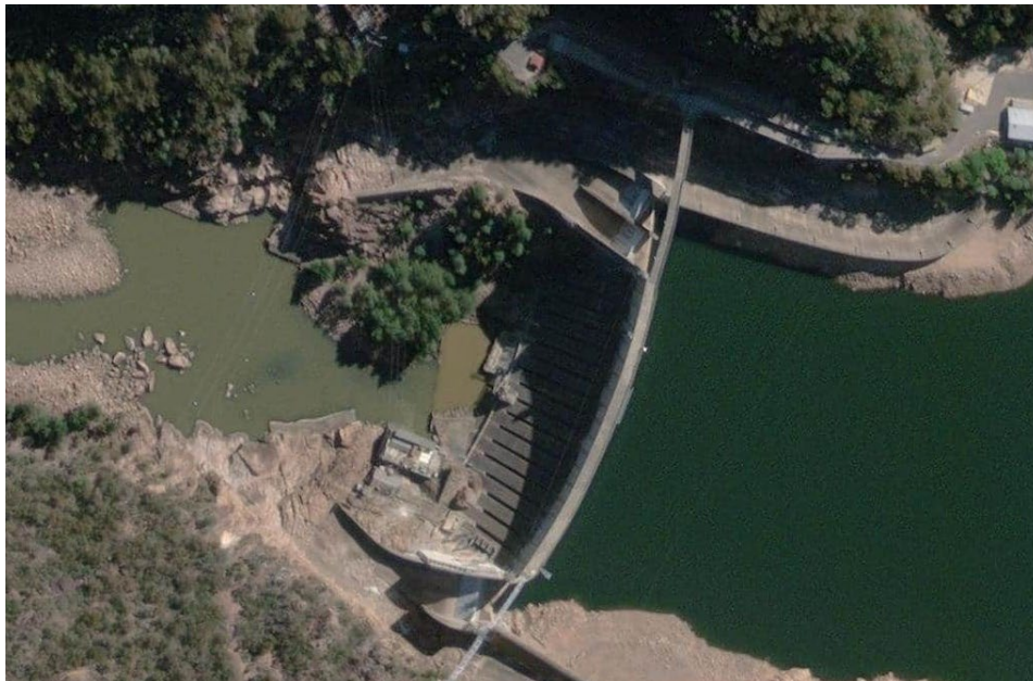
Figure 4.1 Aerial view of Burrinjuck Dam. (Source: Nearmap)
