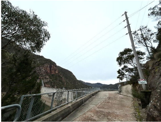
Figure 4.11 Northern aerial conductor cable fixing pole, with the 4 aerial conductor cables attached. (Source: WaterNSW, July 2025)
