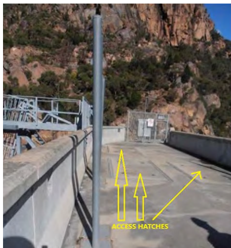
Figure 18: Three access hatches above the Southern Crest Chamber
