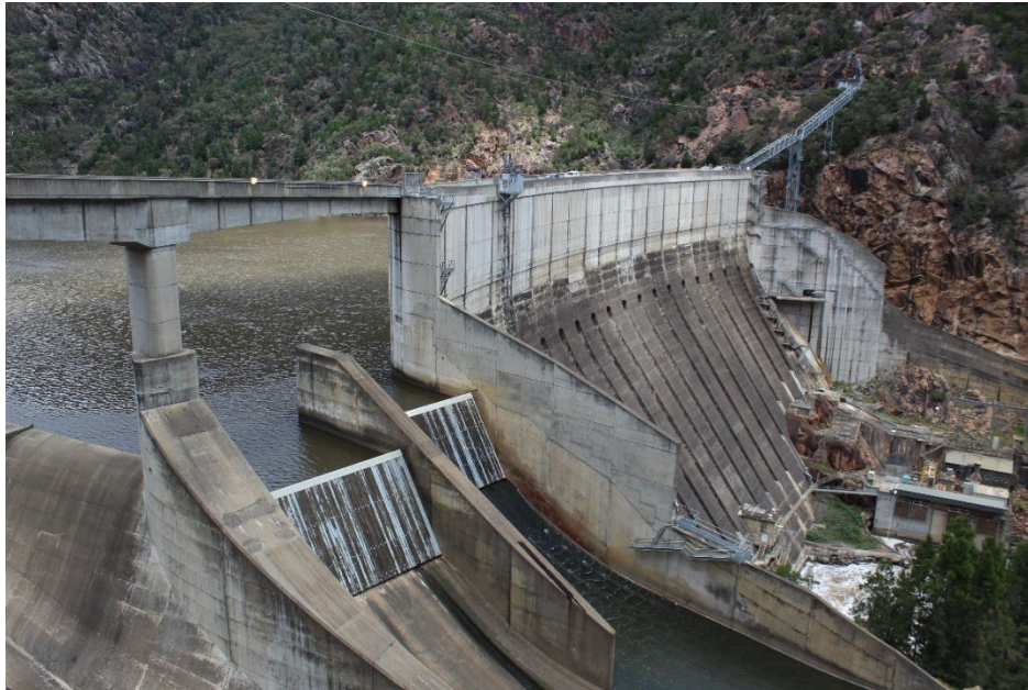
Figure 4.2 View of Burrinjuck Dam from the northwest, 2022. (Source: GML Heritage)
