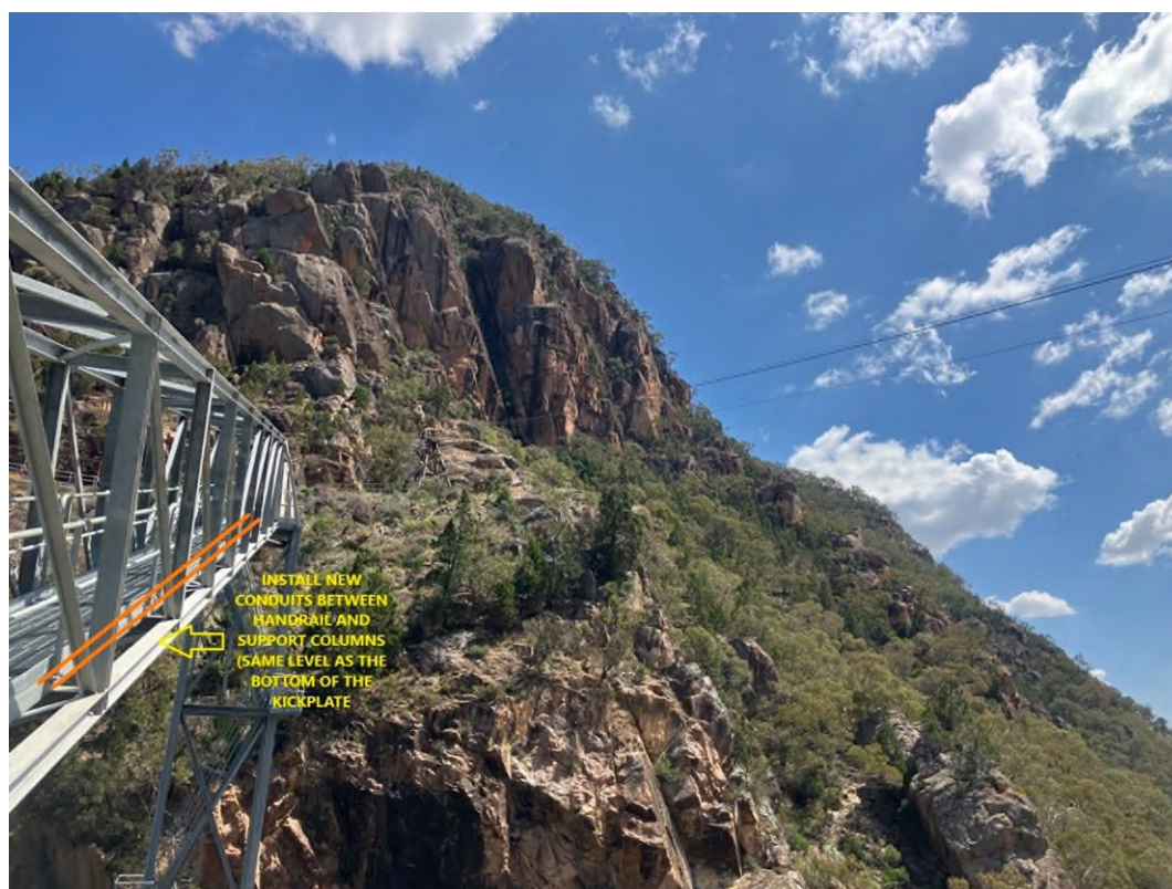
Figure 20: Conduits running parallel to walkway up to the middle landing
