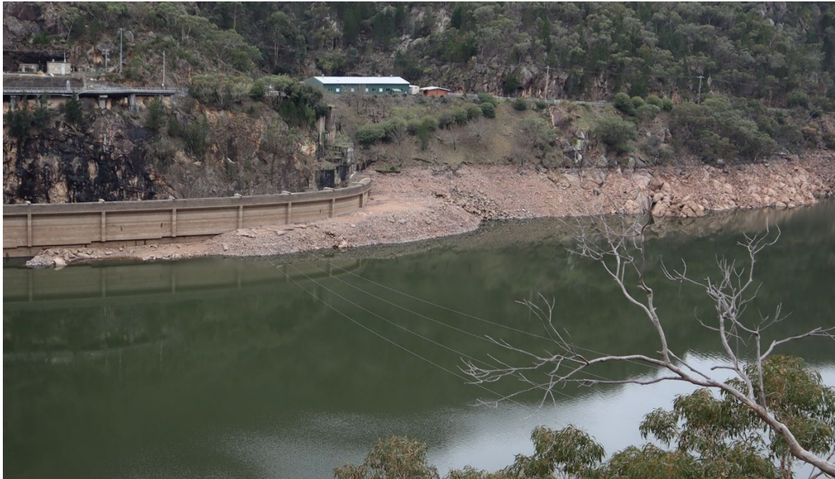
Figure 4.15 Aerial conductor power supply cables between north and south side of dam. (Source: WaterNSW, 2025)
