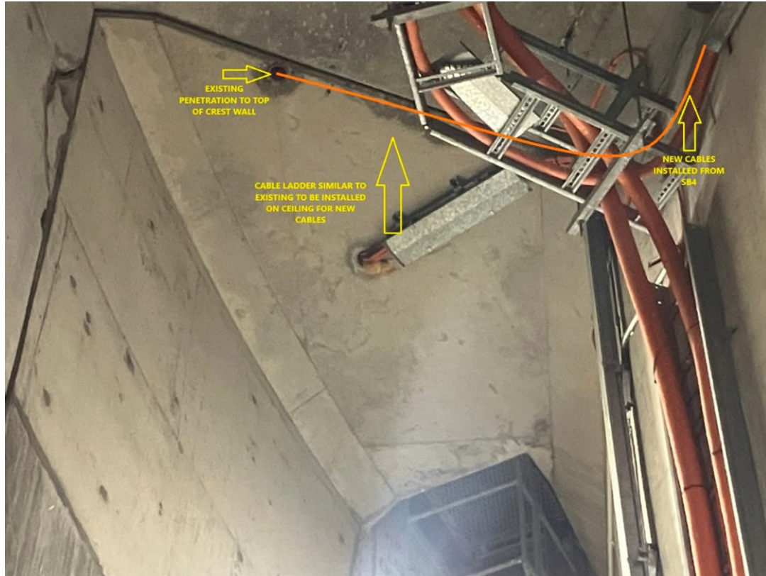
Figure 17: New cable route in the Southern Crest Chamber
