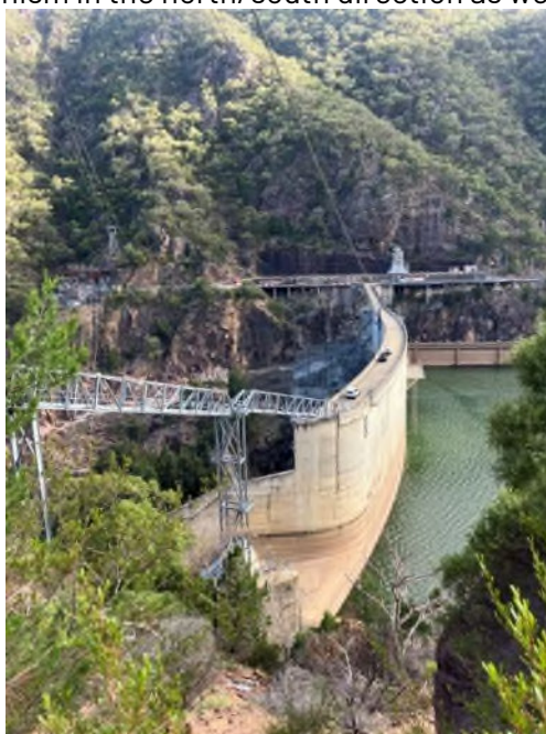
Figure 2: Head/North Tower (white structure)
