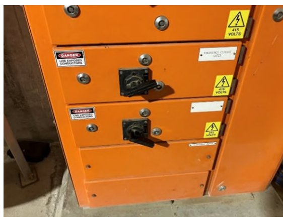
Figure 12: Hydraulic Unit Supply and Spare
