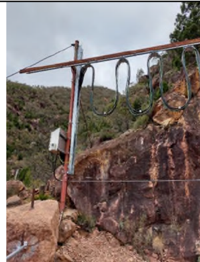
Figure 7: Tail (South) Tower Isolator
