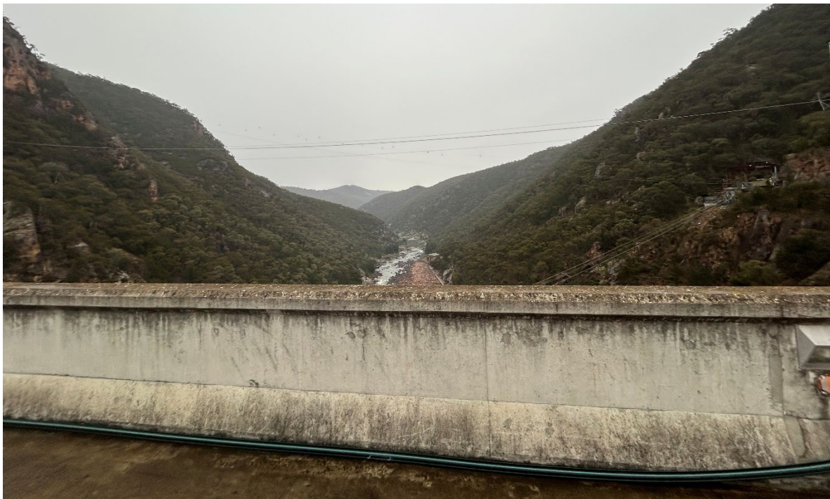
Figure 4.10 Cable between head and tail tower, looking downstream. (Source: WaterNSW, 2025)
