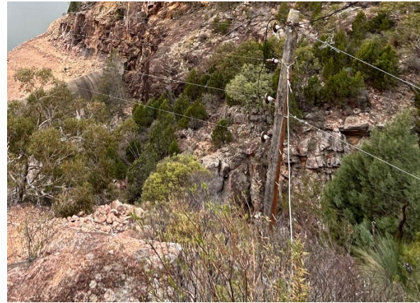
Figure 4.12 Southern aerial conductor cable fixing pole. (Source: WaterNSW, 2025)
