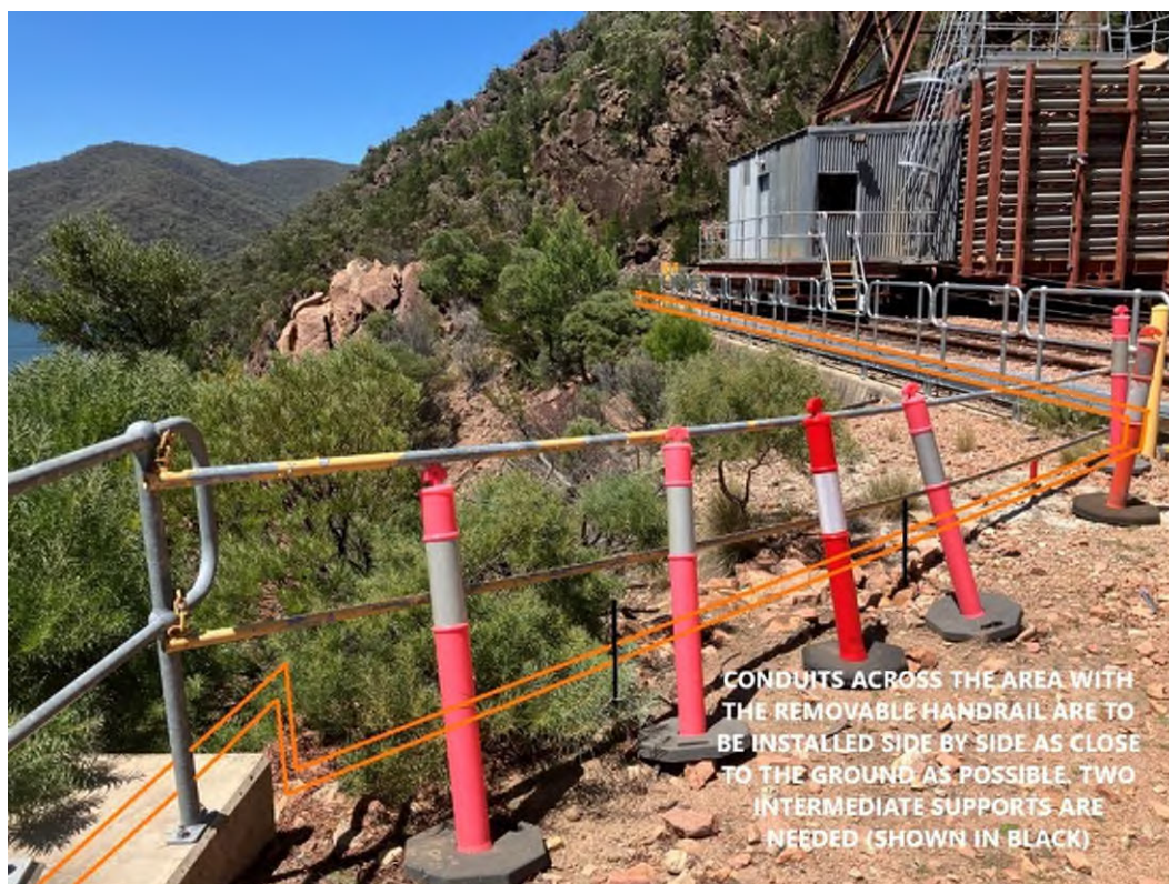
Figure 24: Conduit installation across removable handrail section
