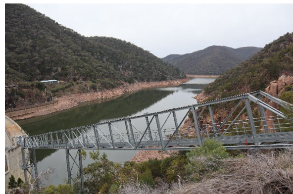
Figure 4.14 Walkway travelling from tail tower platform to dam crest wall. (Source: WaterNSW, July 2025)
