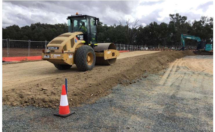
Loading material and earth compaction works for trial embankment, adjacent to Lake Cargelligo Road.
