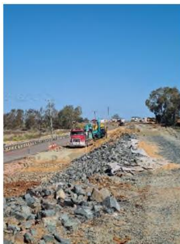
Left: A1 works on Embankment B
