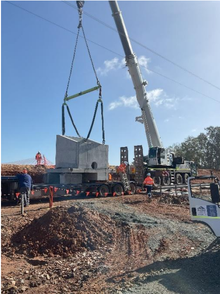
Left: Pit installation at Embankment B Below: Completed Embankment B
