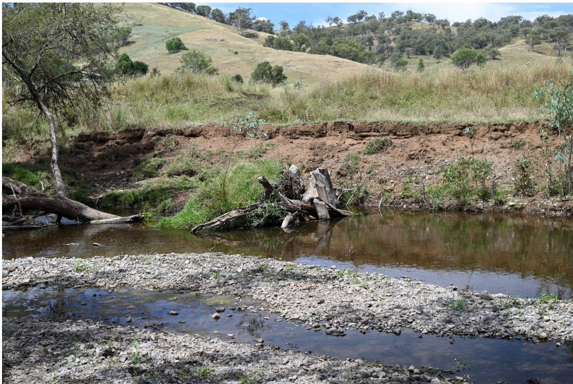
Appendix Photo 2: Engineered snag with collected debris following high flows further enhancing habitat
