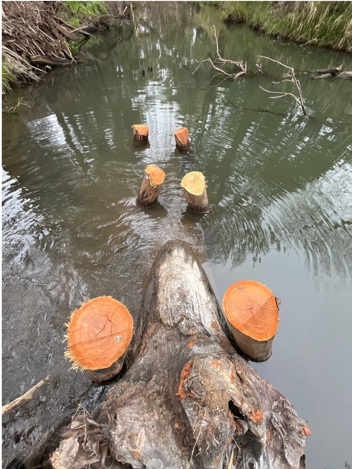
Photo of a typical installed snag and anchor pin logs
