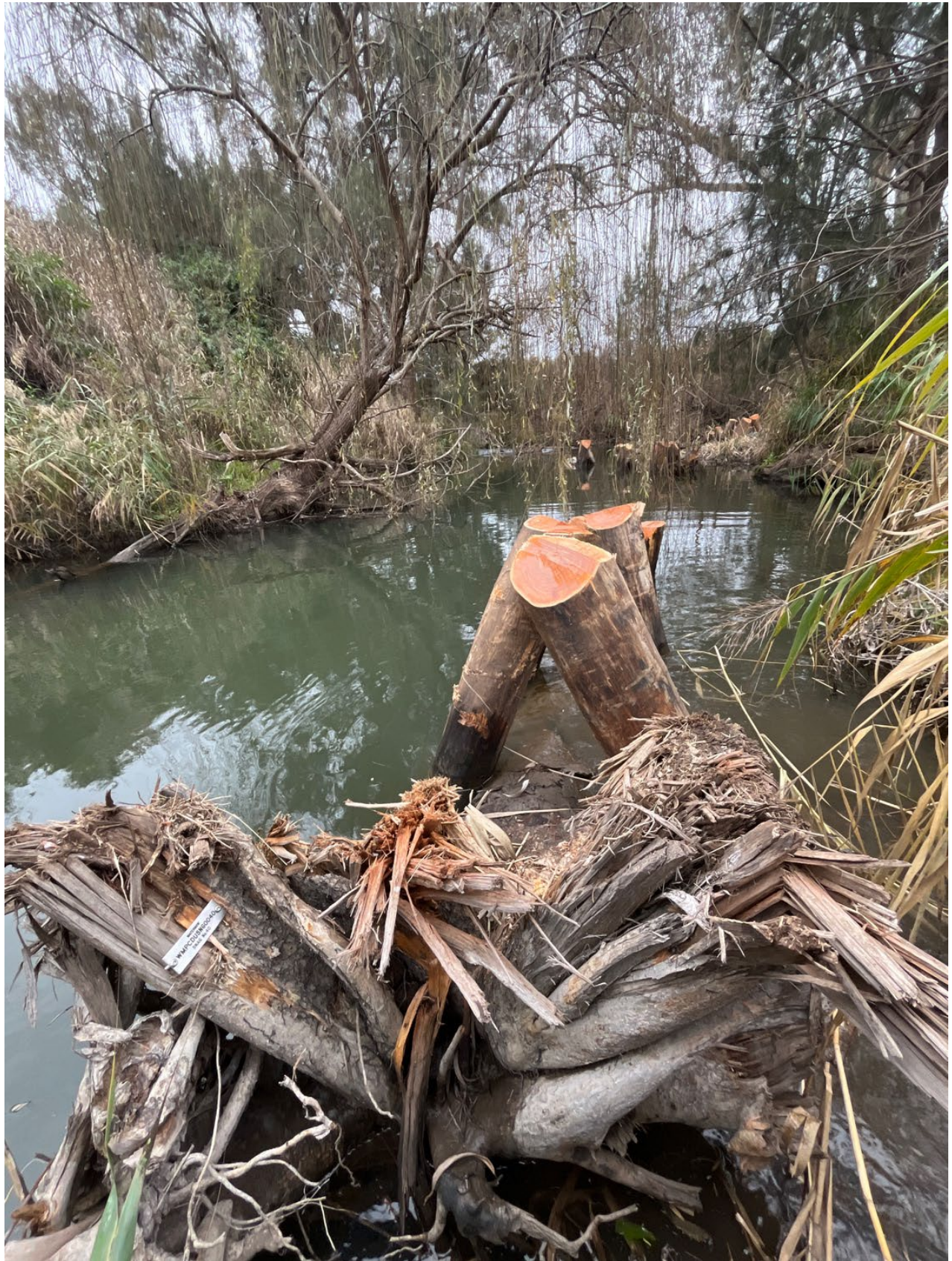
Photo of installed snag with additional installed snag downstream in the stretch of river
