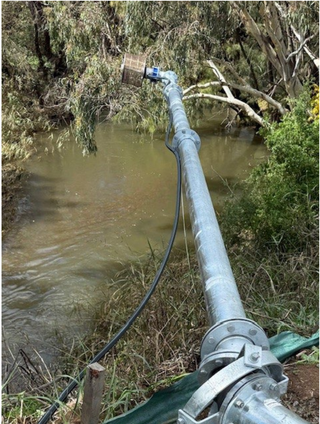
Photo of Installed Self-cleaning pump screen and pump intake and retrieval system on the Peel River
