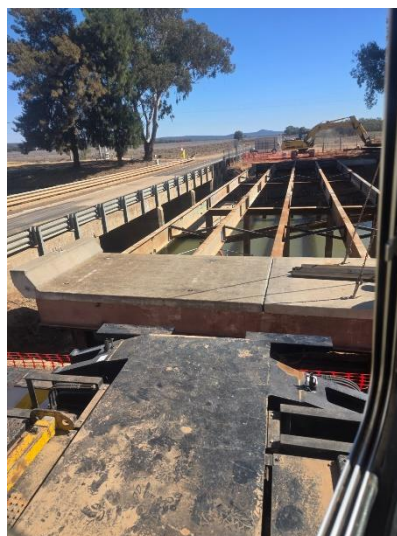
Concrete bridge deck for temporary bridge
