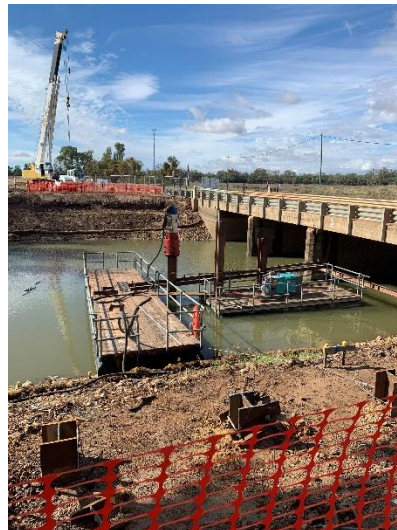
Air hammer driving piles from floating work platform
