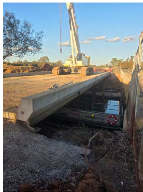
Partially completed temporary bridge
