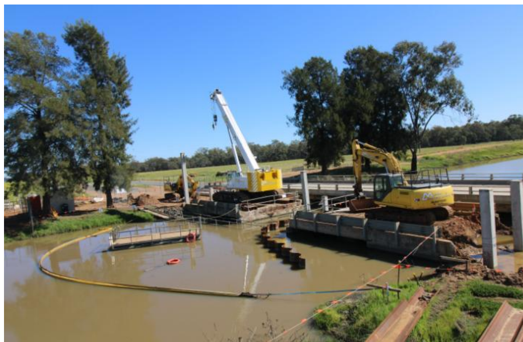
High water levels in the Lake Brewster Inlet Channel causing delays to the replacement of the Ballyrogan Bridge
