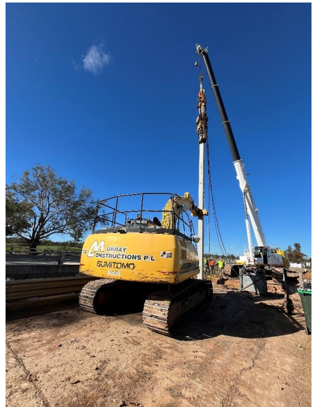
Commencement of pile driving works
