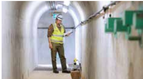
^ AN INSPECTION GALLERY INSIDE WARRAGAMBA DAM
