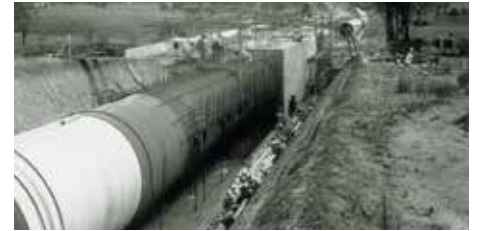
^ CONSTRUCTION OF WARRAGAMBA-PROSPECT PIPELINE, FEB 1966
