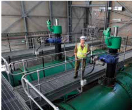
^ THE VALVE HOUSE, WARRAGAMBA
