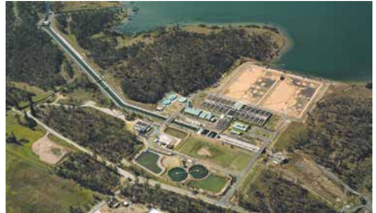
> AERIAL VIEW OF PROSPECT RESERVOIR
