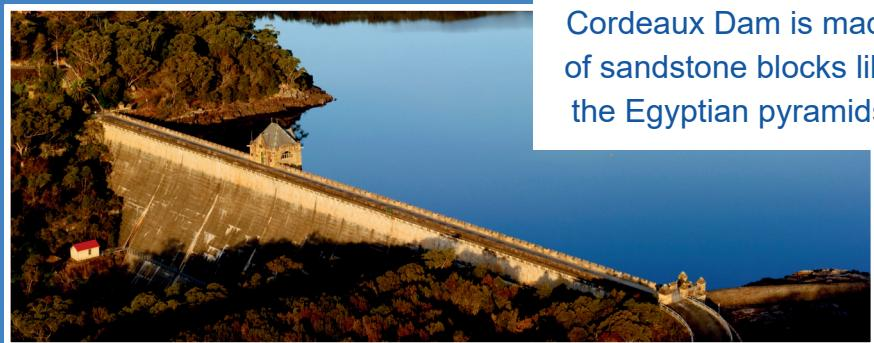
Cordeaux Dam is made of sandstone blocks like the Egyptian pyramids.
