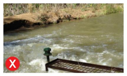
An example can be seen in the picture above of an old walkway to a meter on a bubbler. It has no handrails and no protective barrier to prevent a fall into the water when reading the meter. There are two available options:
