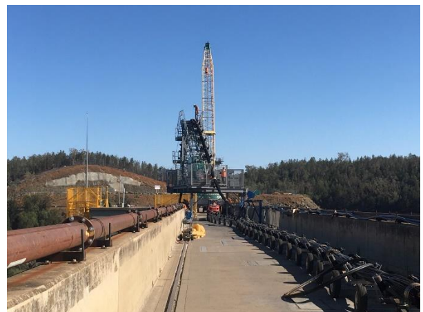
Photo: Keepit Dam installation of spillway pier anchor
