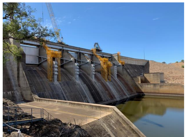
Photo: Keepit Dam spillway and gates
