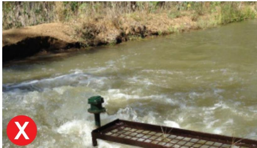
An example can be seen in the picture above of an old walkway to a meter on a bubbler. It has no handrails and no protective barrier to prevent a fall into the water when reading the meter. There are two available options:
