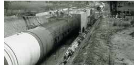
^ CONSTRUCTION OF WARRAGAMBA-PROSPECT PIPELINE, FEB 1966
