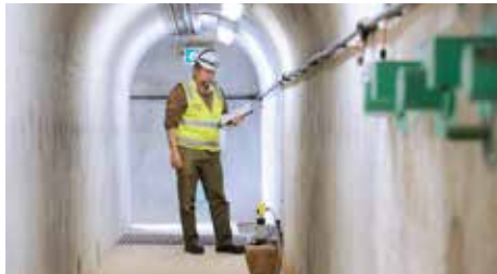
^ AN INSPECTION GALLERY INSIDE WARRAGAMBA DAM
