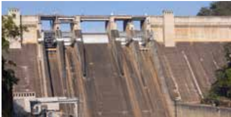
^ WARRAGAMBA DAM WALL
