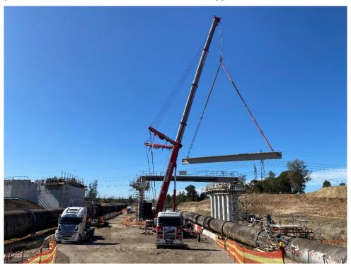
Figure 21 – bridge girder suspended over the dewatered pipeline at Erskine Park
