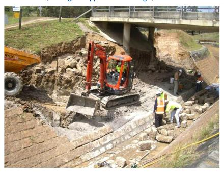
Figure 20 - Reconstruction of Upper Canal wall collapse (2008)
