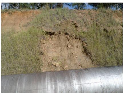
Figure 19 - Embankment slippage along the Warragamba Pipelines Corridor
