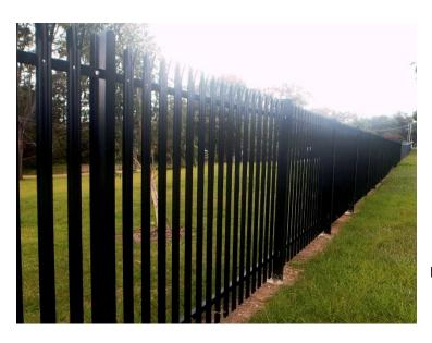
Figure 13 - Palisade fencing
