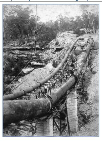
Figure 26 - Leafs Creek Aqueduct sometime between 1886 and 1888 showing the temporary Hudson's scheme aqueduct
