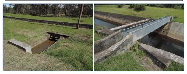
Figure 22 – Examples of Upper Canal drainage systems (left – culvert, right – steel box flume)
