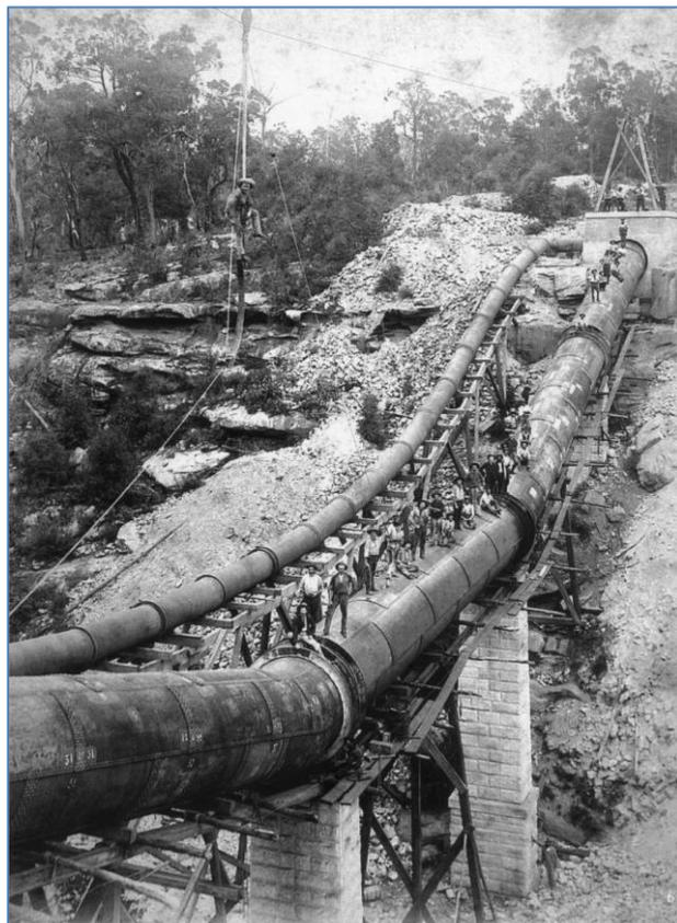
**Figure 26** - Leaf Creek Aqueduct sometime between 1886 and 1888 showing the temporary Hudson's scheme aqueduct
