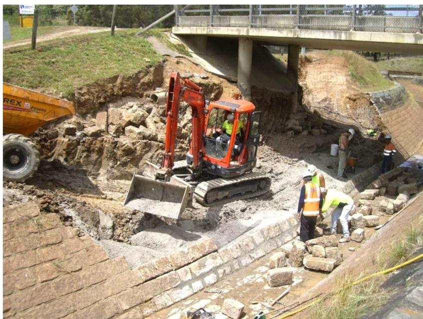
**Figure 20** - Reconstruction of Upper Canal wall collapse (2008)
