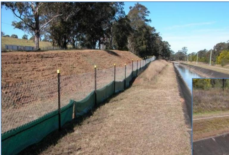
**Figure 23** – Examples of suitable erosion control adjacent to the Upper Canal
