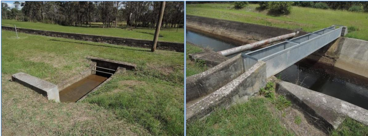
**Figure 22** – Examples of Upper Canal drainage systems (left – culvert, right – steel box flume)
