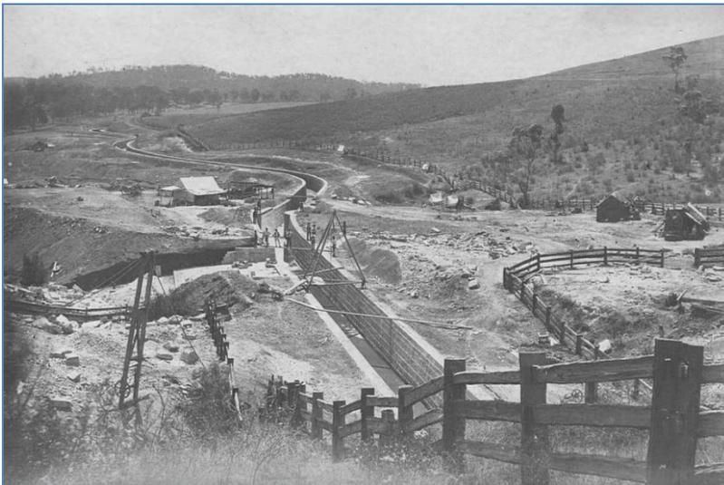
**Figure 24 (left)** – The Upper Canal during construction in the 1880s north of Sugarloaf Hill
