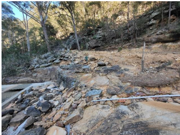
Current condition of the weir access track
