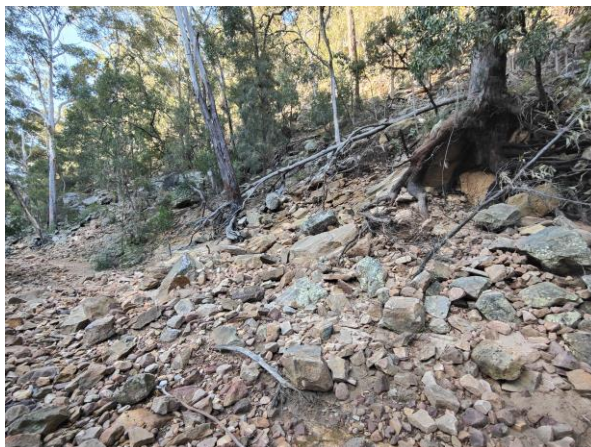
Landslide blocking access to the weir
