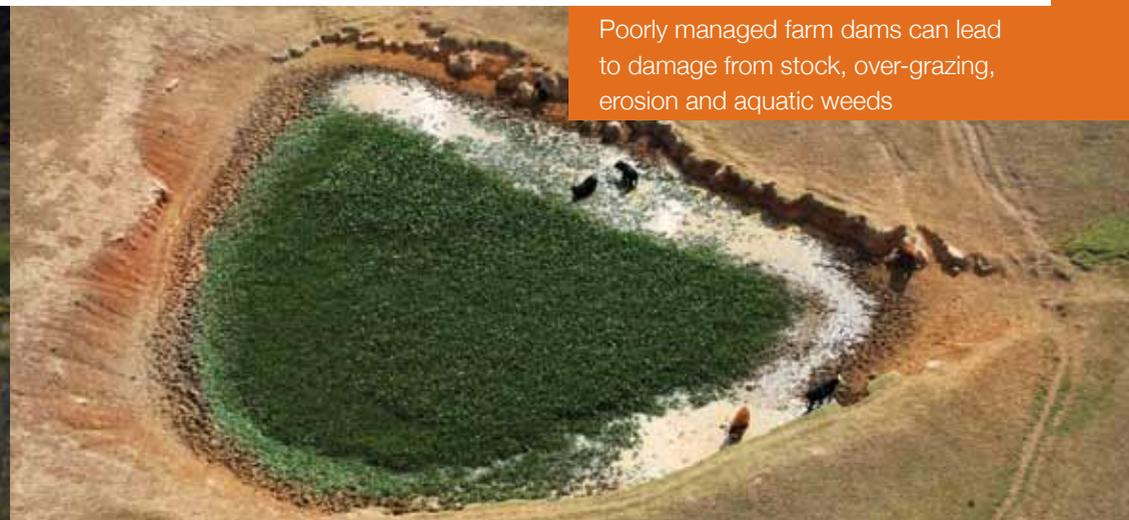
Poorly managed farm dams can lead to damage from stock, over-grazing, erosion and aquatic weeds
