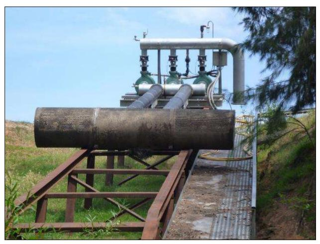
Figure 40. Example of a pump with screen on the Lachlan River
