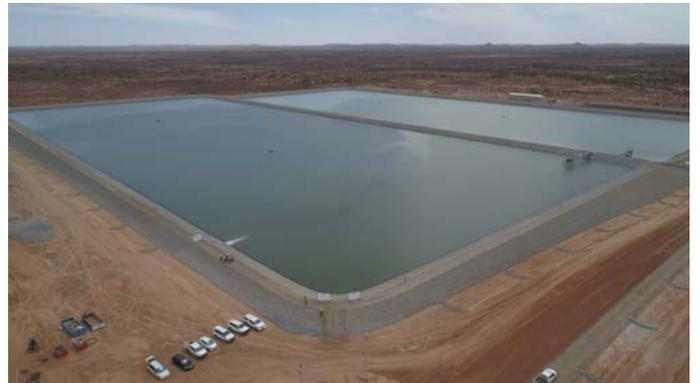
An important part of the W2BH Project is the 720 megalitre bulk water storage built on the outskirts of Broken Hill. The storage will ensure constant water supply during pipeline maintenance periods.
