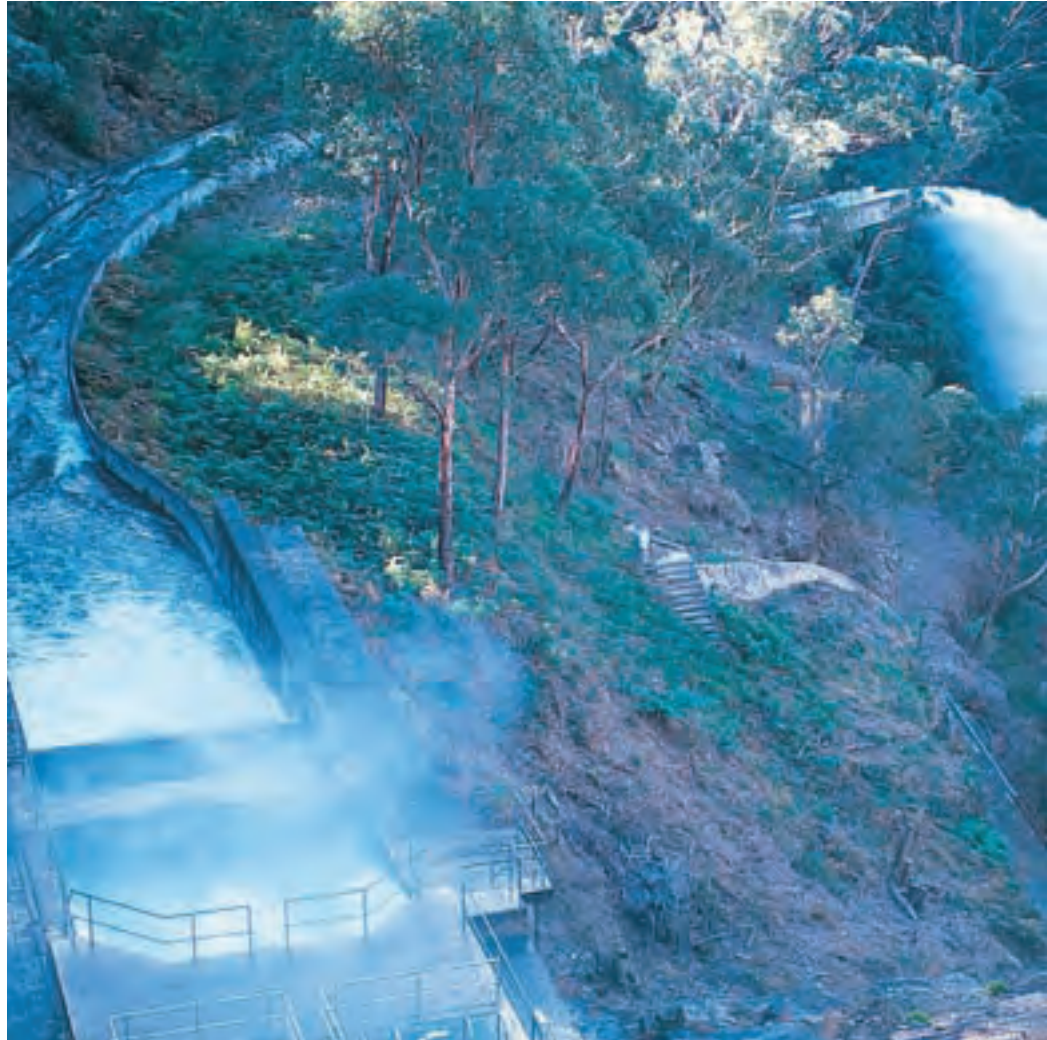
→ AVON DAM DISCHARGE CHUTE
