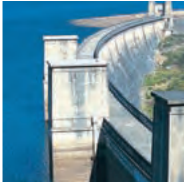
← CURVED WALL OF CORDEAUX DAM
