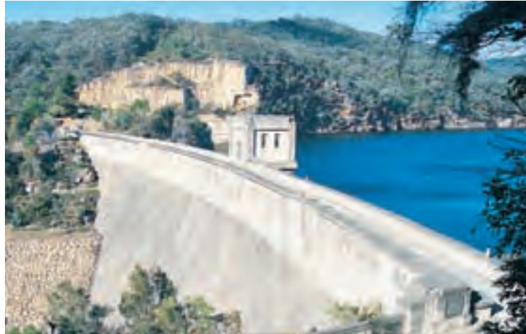
↑ MASSIVE SANDSTONE BLOCKS USED IN DAM WALL CONSTRUCTION ← NEPEAN DAM
