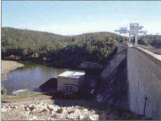
Figure 4.2 Keepit Dam Wall
