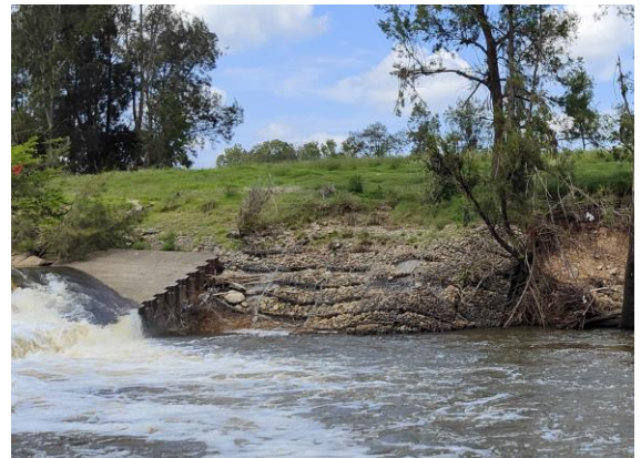
Camden Weir before the erosion repairs
