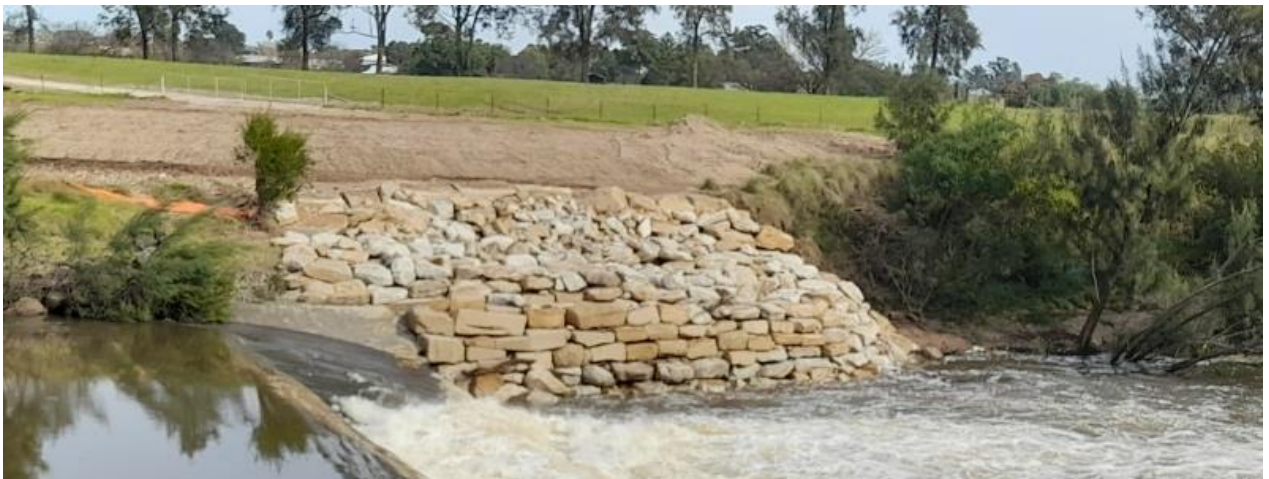
Camden Weir after the erosion repairs
