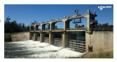
environmental factors, extending their life by up to 25 years. This will enable WaterNSW to provide continued service to customers, including management of water diversion in to Mehi river. The work follows routine maintenance which identified a need to address corrosion and deterioration of the metal gates
