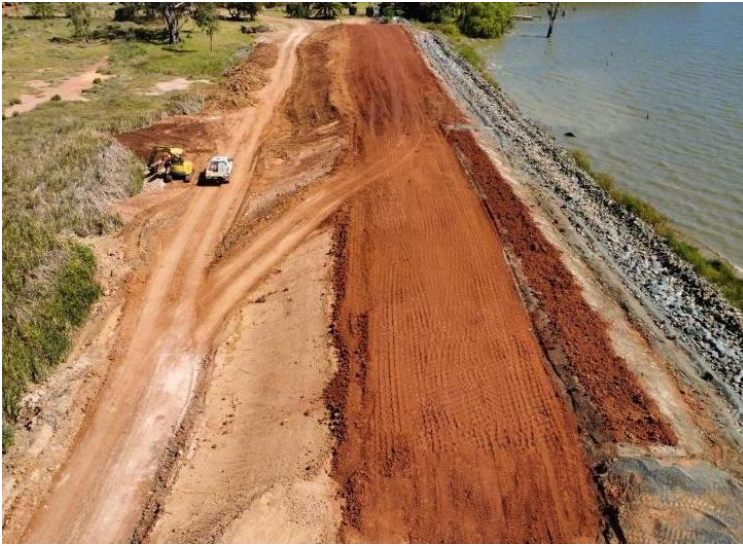
Clay placement on Embankment C2
