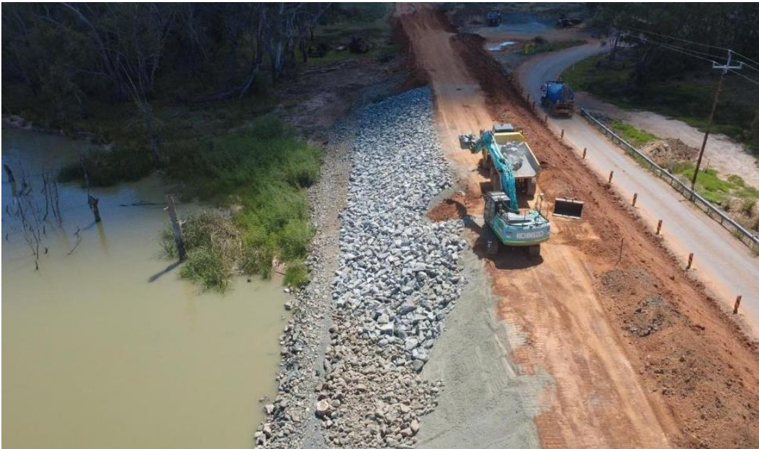
Clay placement on Embankment C2
