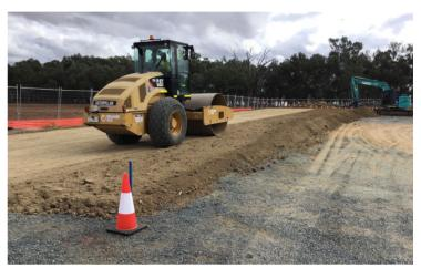
Loading material and earth compaction works for trial embankment, adjacent to Lake Cargelligo Road.
