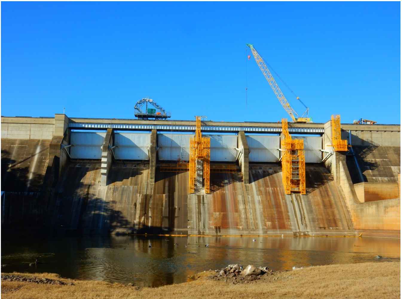
Figure 1 – Dam wall from downstream
