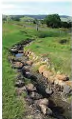
Rock lined drainage treatment
