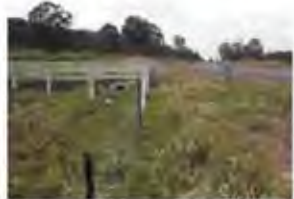
Driveway: Stormwater culvert
