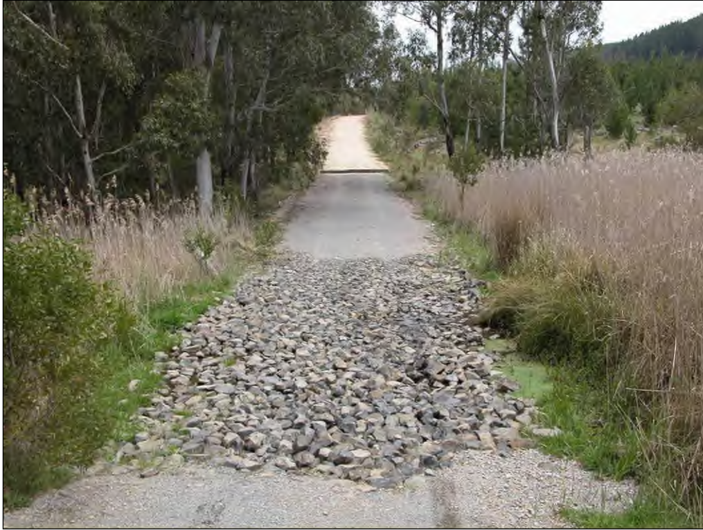
Figure 3-9 Water sensitive watercourse crossing showing a diversion, gravel and large rocks to allow flow
