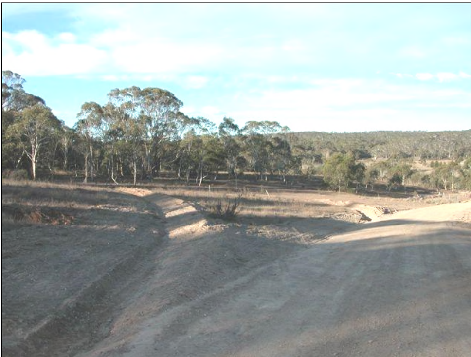
Figure 3-6 Unsealed road showing two recently constructed mitre drains
