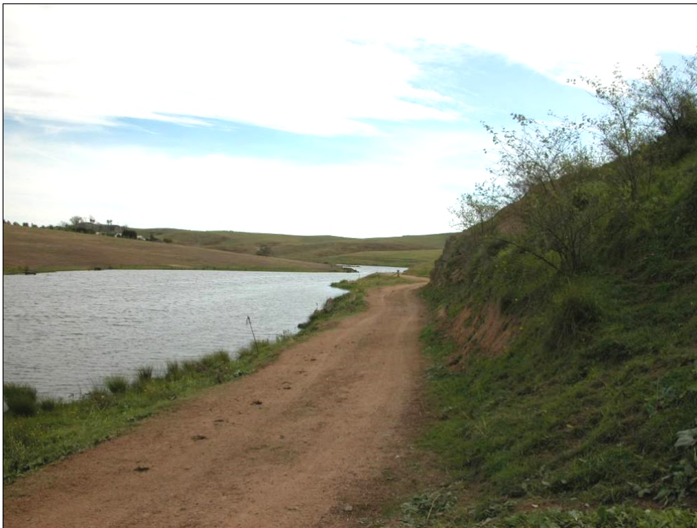
Figure 3-5 Construction of this road required large amounts of cut and fill, and is too close to the waterway
