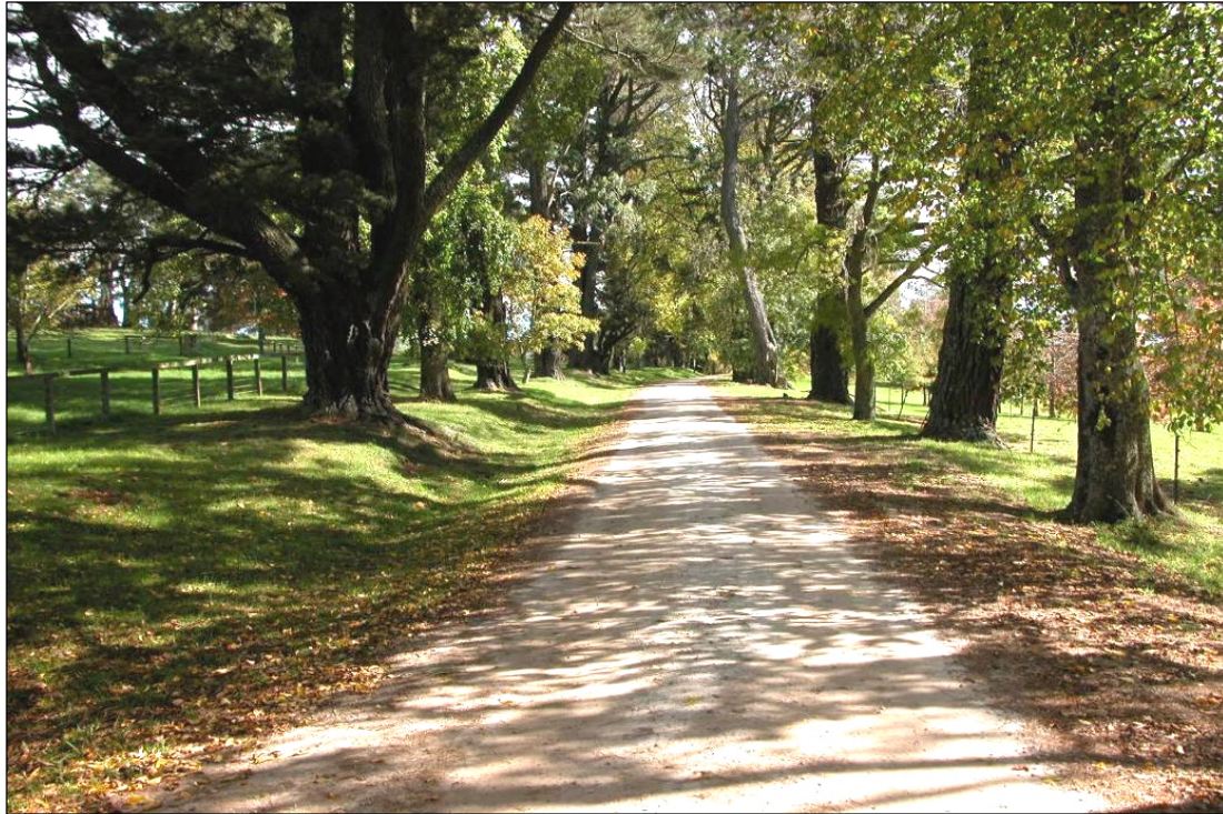
Figure 2-10 This existing access-way would be an asset to a subdivision because of its satisfactory cross fall and grassed drainage swale
