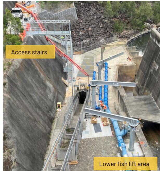
New stairs and ladders make it safer for workers to access the site and maintain the fish lift. New cranes help safely lift and move heavy equipment during maintenance work. We've also replaced pipes, valves and screens in the lower fish lift area.
