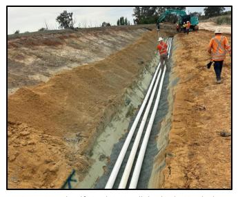
$Drainage\ pipework\ and\ fittings\ being\ installed\ within\ the\ C2\ embankment$
