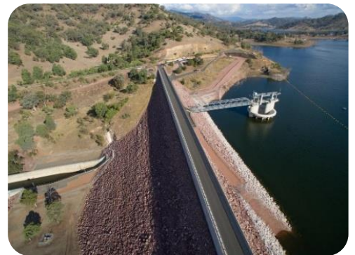
Chaffey Dam is a rock-fill dam with a clay core. The rock wall is 443 metres long and 55.8 metres high.
