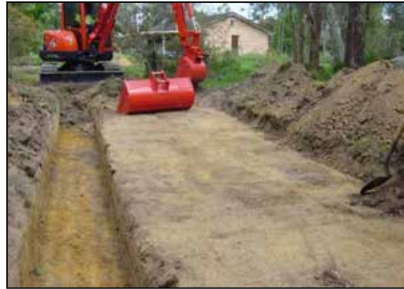
Figure 10.14 and 10.15 Excavation of the bed of the “Wick” trench
