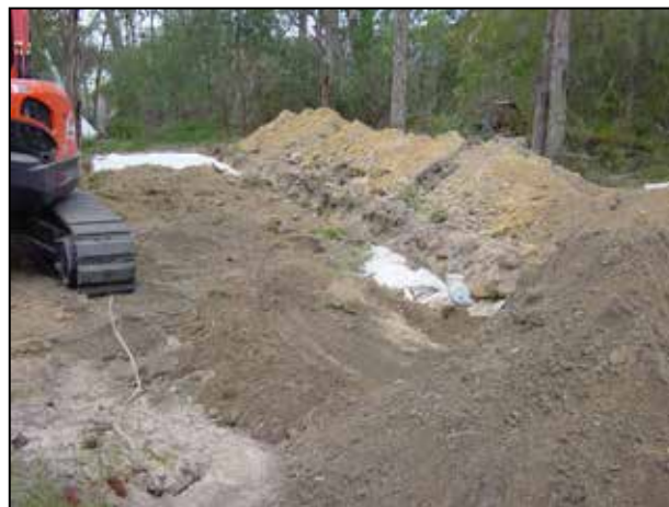
Figure 10.20 Backfilling and the inspection ports
