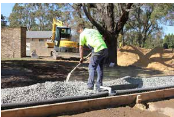
Figure 9.5 Gravel over inlet manifold
