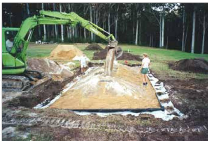
Figure 8.7 Final shaping of cell mound
