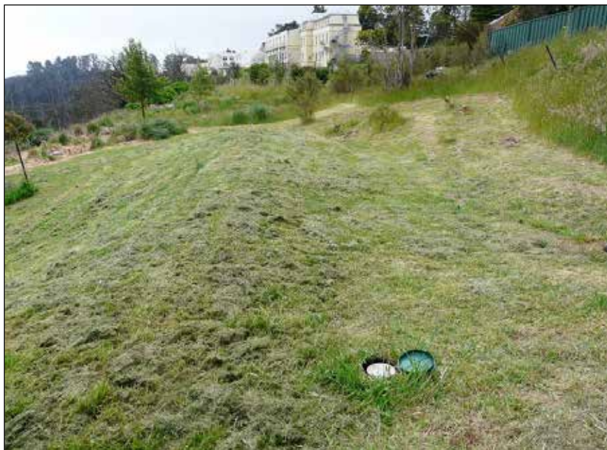
Figure 8.1 An amended soil mound in the Blue Mountains
