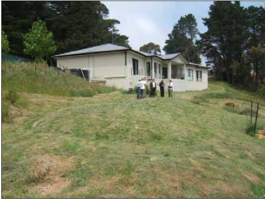
Figure 8.9 Amended soil mound constructed on sloping site
