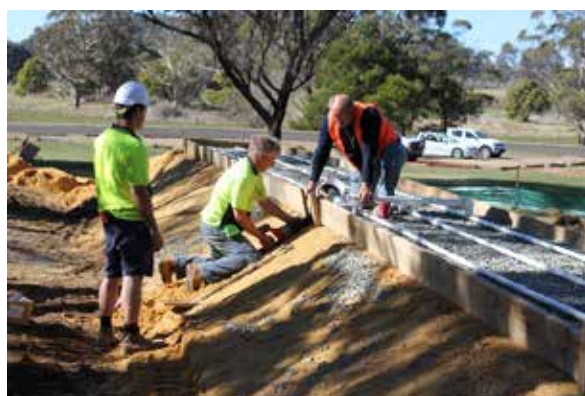
Figure 9.4 Constructing the manifold
