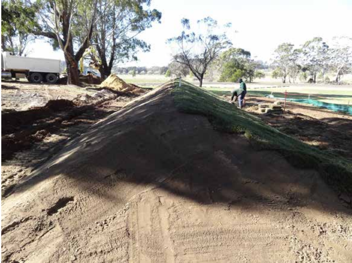
Figure 9.7 Turfing the mound
