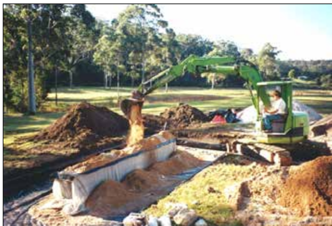
Figure 8.6 Backfilling with amended soil
