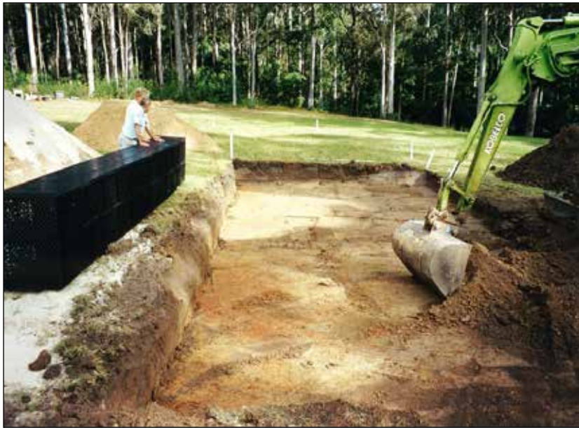
Figure 8.3 Excavation/preparement of base of mound (Figures 8.3-8.7 Ecomax, 2001)
