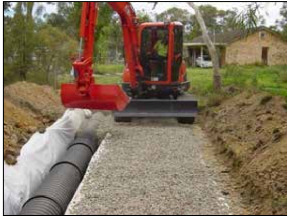
Figures 10.18 Backfilling gravel layer
