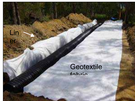
Figure 10.16 and 10.17 Laying the liner in the trench and then the geotextile fabric as the ‘wick’ across the pan
