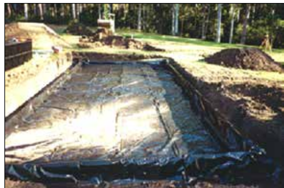
Figure 8.5 Lining with an impervious liner
