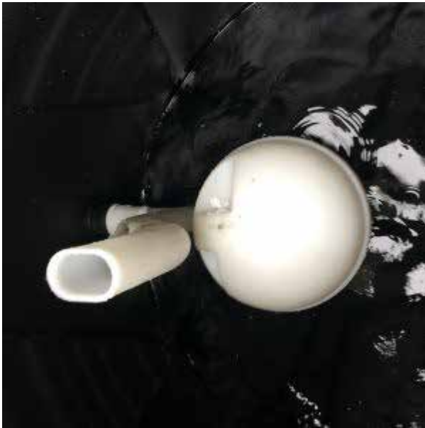
Figure 14.2 Dosing siphon in dosing chamber (Surge-flow 100)
