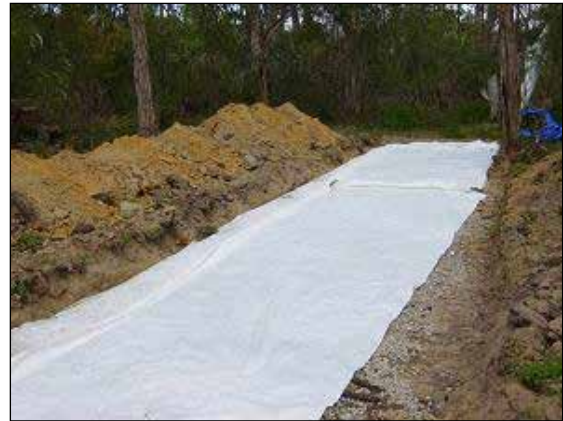
Figure 10.19 Adding the second geotextile fabric layer
