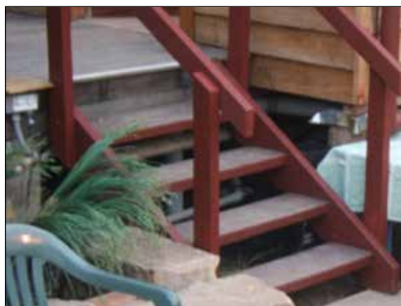
Figure 6.4 New steps blocking access to the composting unit
