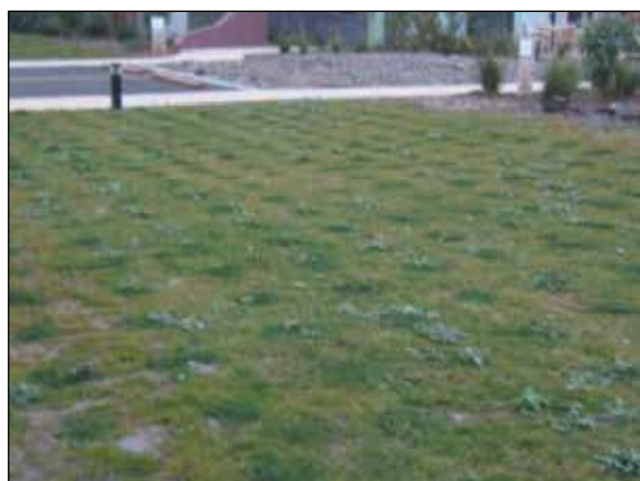
Figure 13.2 An installed subsurface irrigation system with close emitter spacing (Whitehead & Associates)
