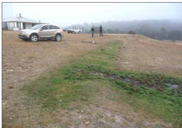
Figure 10.10 Failing trench
