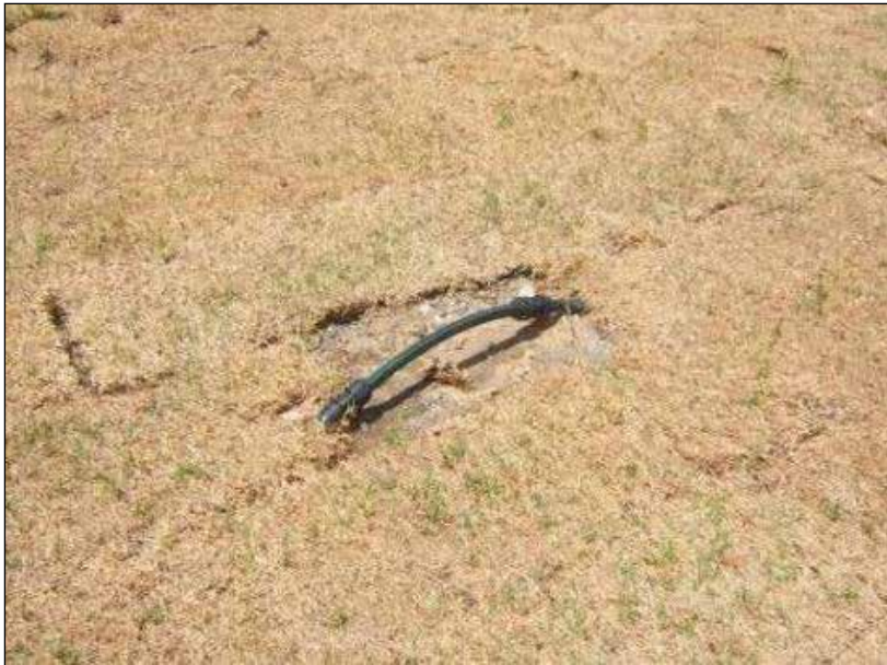
Figure 13.7 Damaged irrigation line sections cut out and replaced as part of an unsatisfactory repair.
