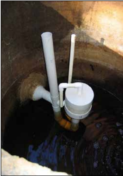
Figure 10.3 Dosing siphon (Arris Wastewater Clinic)
