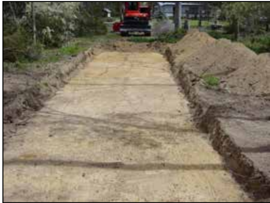
Figure 10.14 and 10.15 Excavation of the bed of the “Wick” trench
