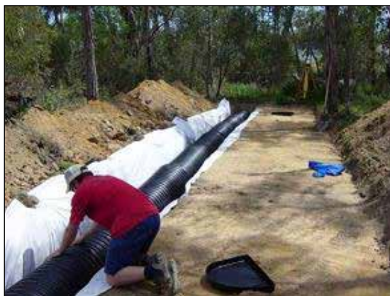
Figure 10.16 and 10.17 Laying the liner in the trench and then the geotextile fabric as the ‘wick’ across the pan
