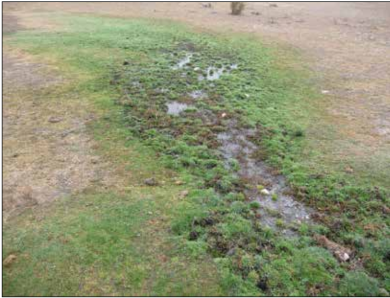
Figure 10.11 Failing trench
