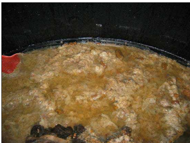
Figure 5.9 A flooded system due to pump failure
