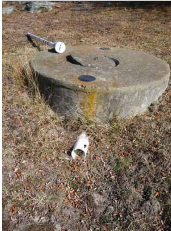
Figure 3.7 Outlet pipe discharging directly onto open ground
