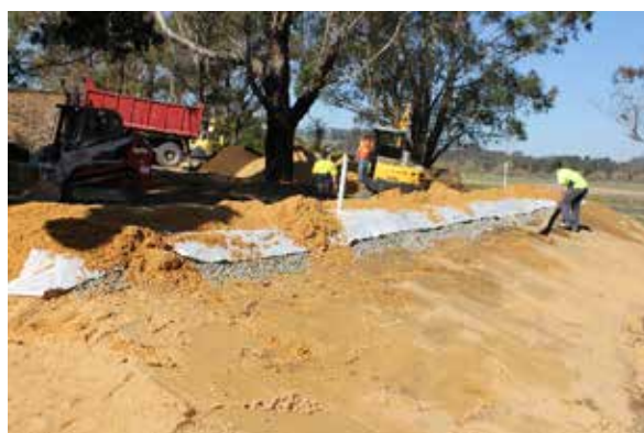
Figure 9.6 Sand on top of geotextile fabric
