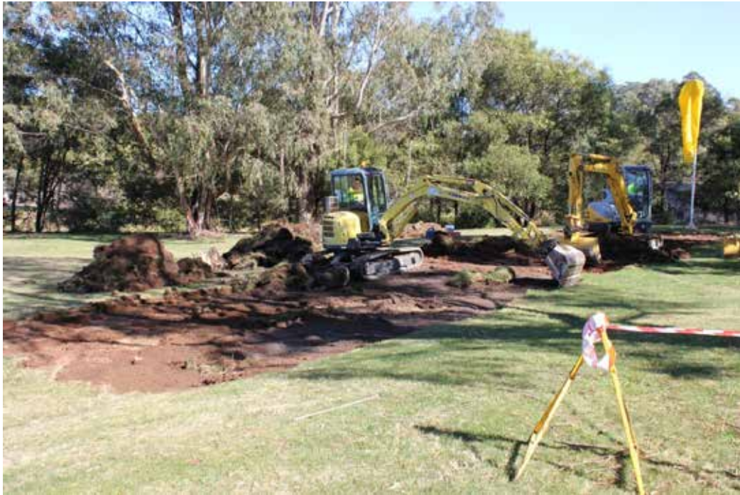
Figure 9.2 Excavation/preparation of base of mound
